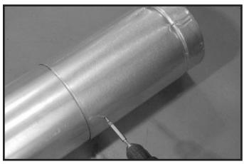
Figure 10.4 Screws into Slip Section
